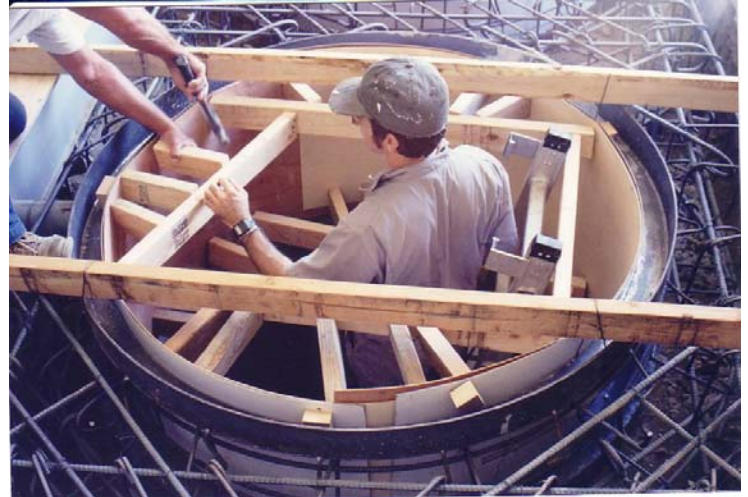
The safest place for cryostats may be underground. Underground vaults from reinforced concrete provide protection against many hazards.
